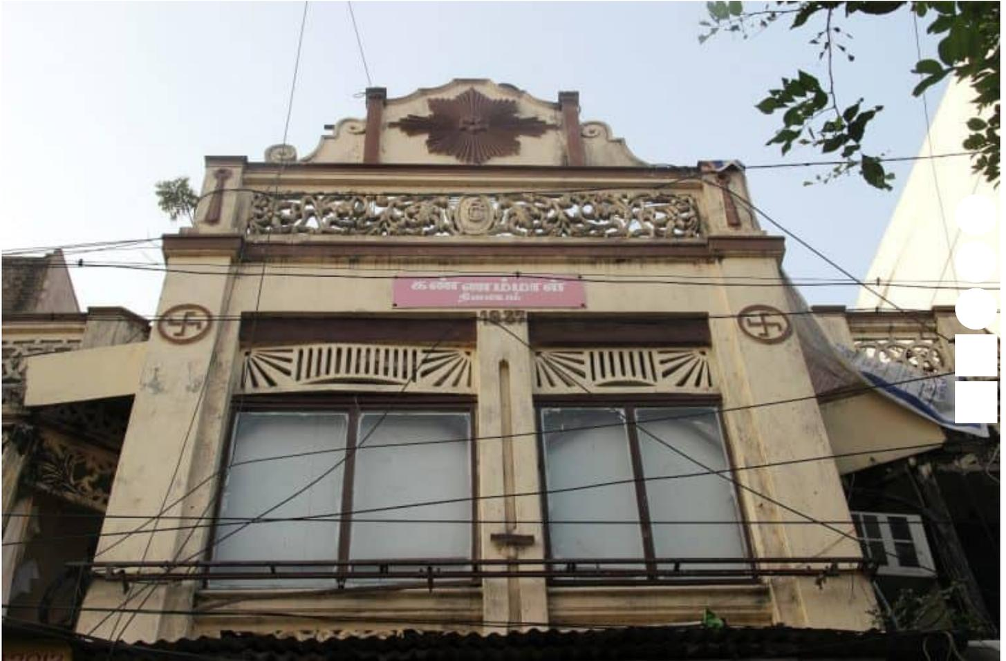
**Straight lines dominated facades; wooden detailing was replaced by concrete. A house with neo-classical influences on South Mada Street, Mylapore.**
